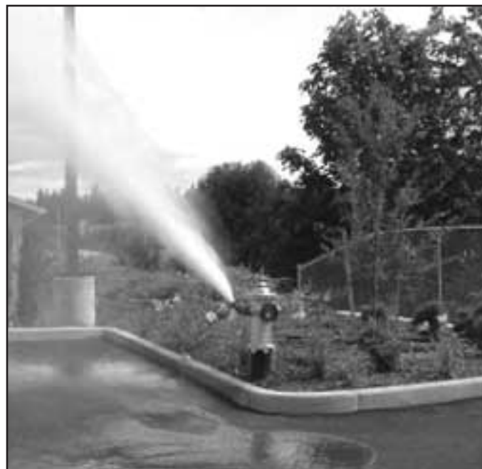
Fire hydrant being flushed.
